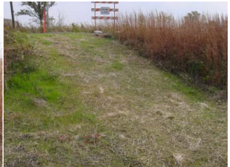
Reseeding after Placement of Fiber Optic Cable
