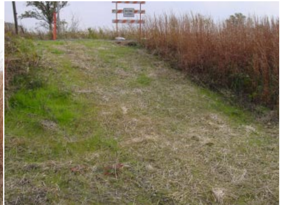
Reseeding after Placement of Fiber Optic Cable
